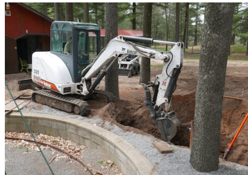
Mike trenching for the conduit to roundhouse.
