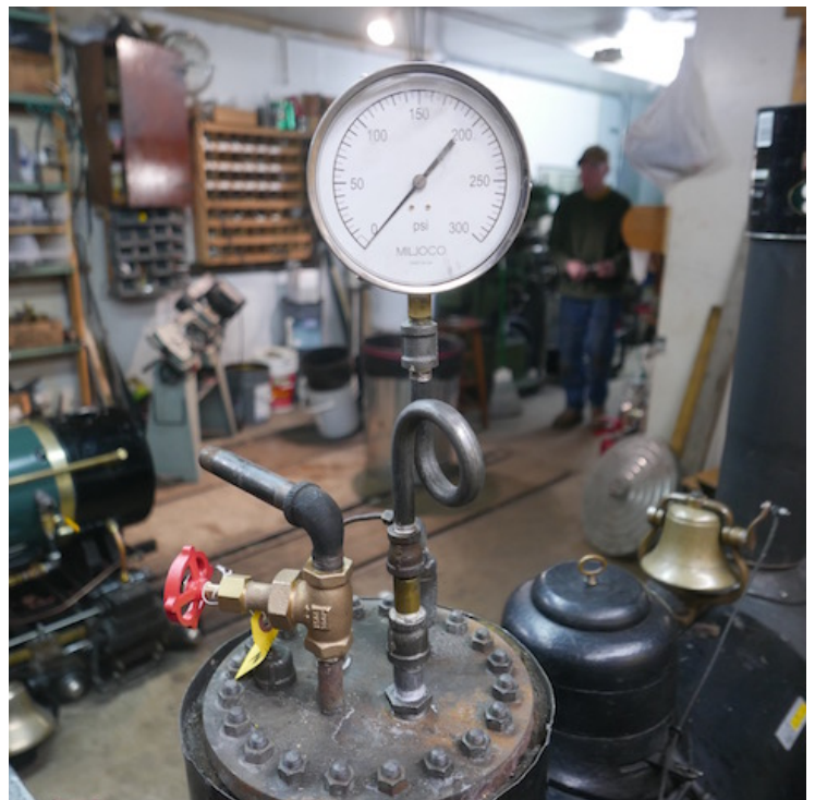
#19 prepped for hydro testing
