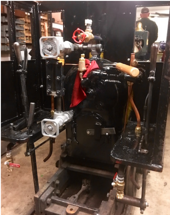
New site glass valves fitted and ready to go
