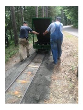
**Track Work** Marc and Chuck operate the dump doors to spread ballast outside of the rails. The dump doors were inspired by the "Tainter" gate design for controlling water at dams. Tainter gates were first used on the Red Cedar River, in Dunn County WI. The gates are still lives on in the dam that holds back the waters of the Red Cedar River, into the old "mill pond," Lake Menomin.
