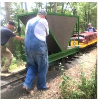
At Lakeside. Ballast as placed at Lakeside. (Near the grade crossing). Two passes with the ballast car spread this material at the sides of the rails. As one can note, much more material than the previous ballast car per trip. Now we can begin leveling and aligning.
