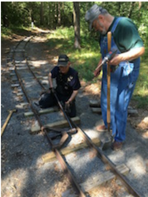
Marc and Chuck removing a slight rail kink with rail bender.
